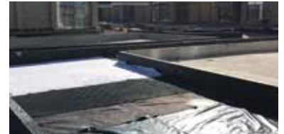
Roof Drainage and Insulation
