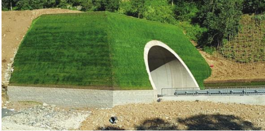
Retaininfg Wall and Steep Slopes
